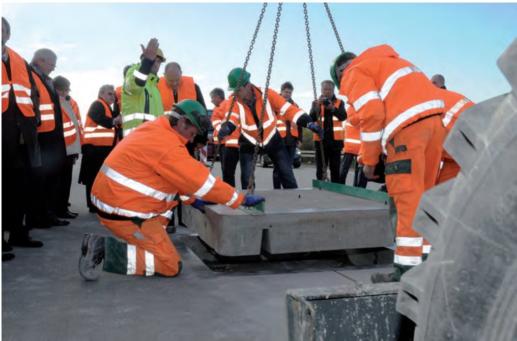
Installation of prefabricated concrete part on the A 9 motorway
