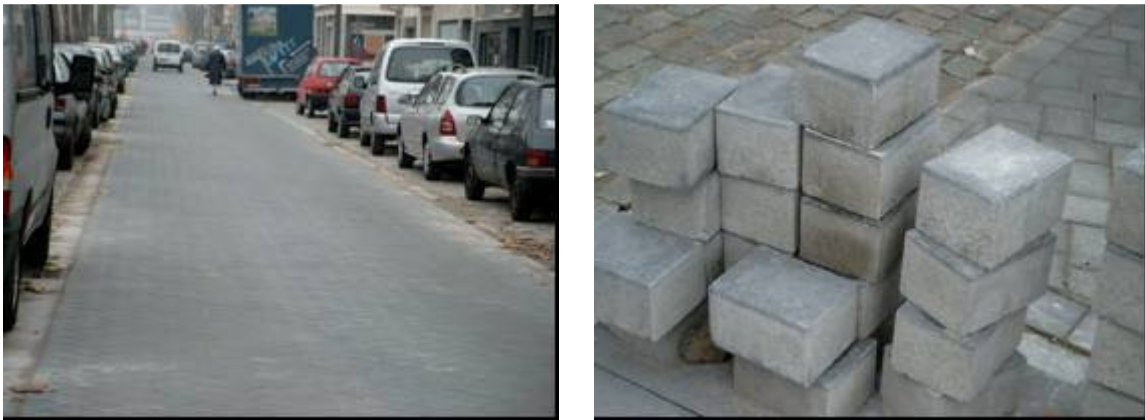
Figure 4 - Separate parking lanes at the Leien of Antwerp with photocatalytic pavement blocks.
