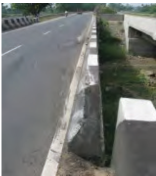
Figure 15. An Open Ended Bridge Wall Built Very Close to the Roadway (left) was the Cause of a Truck Crash; and a Crashed Car which Impacted the Concrete Poles (right).
