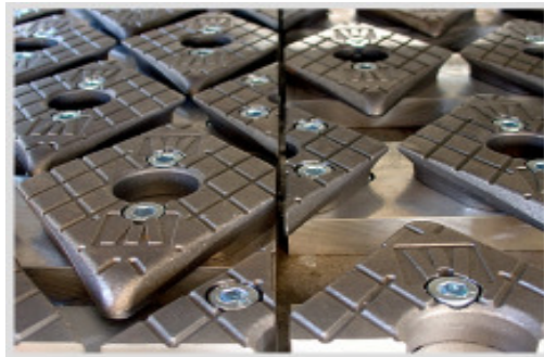
Figure 10: Surface modification of expansion joints to reduce noise emission. left: summer and right: winter expansion
