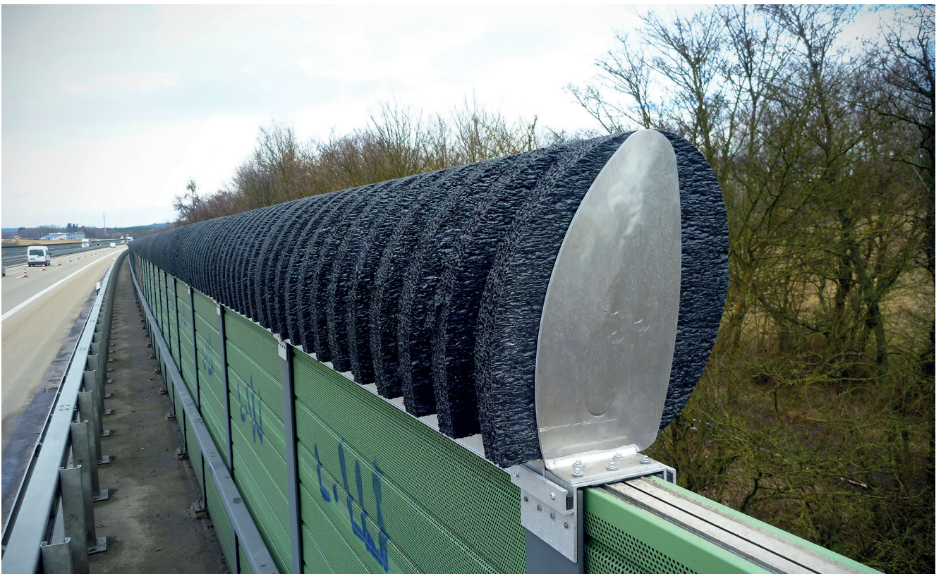
Noise-reducing extension made of whisper foam on top of a noise barrier (photo: Andre Jaborek, Hessen Mobil)
