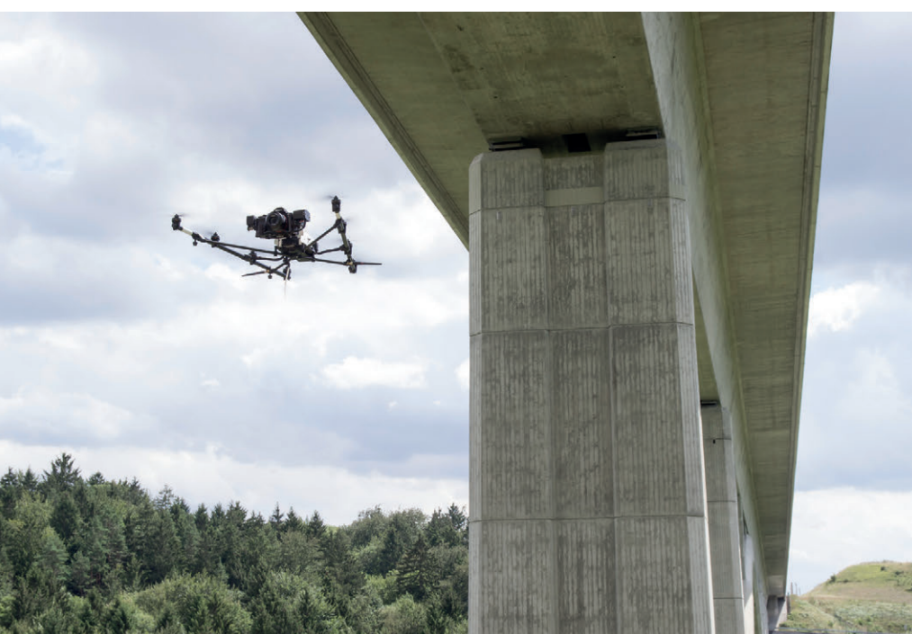
UAS at a bridge structure (photo: gmtib)
