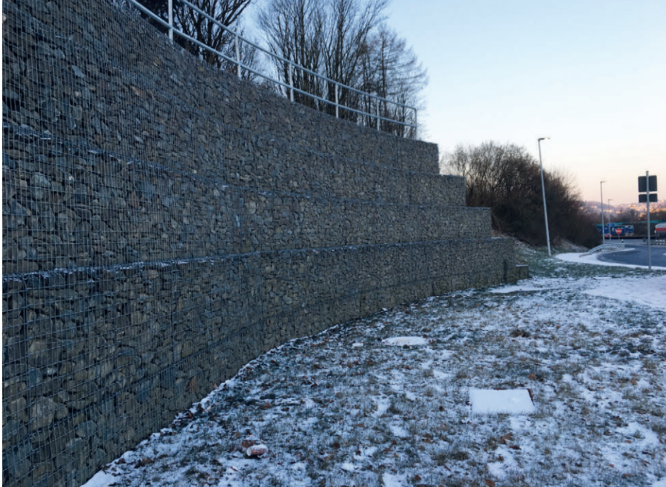
Retaining wall made of gabions
