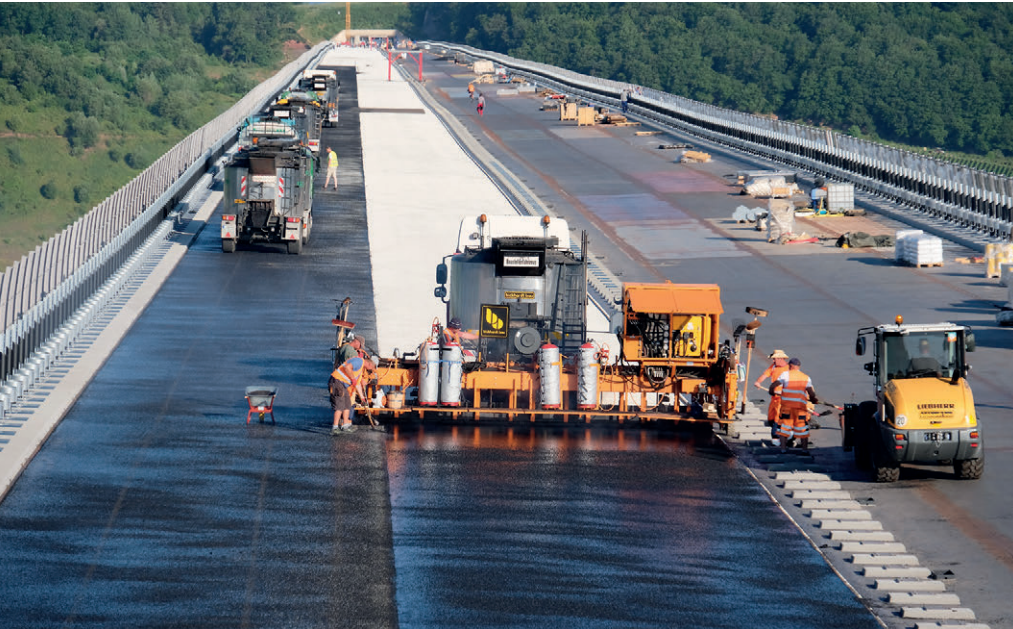
Installing a protective mastic asphalt layer on 28 June 2019
