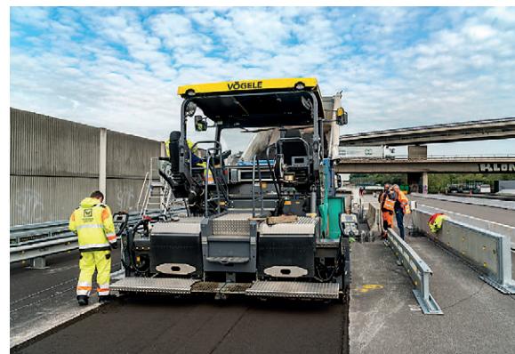
Installation process of a Cold Recycling layer on duraBAST
