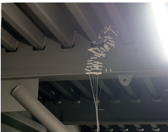
Positioning of temperature sensors inside the bridge at cross beam No. 6
