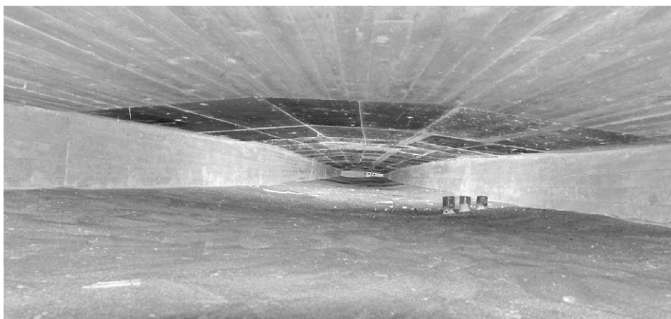
Point cloud from the laser scan in the box girder
