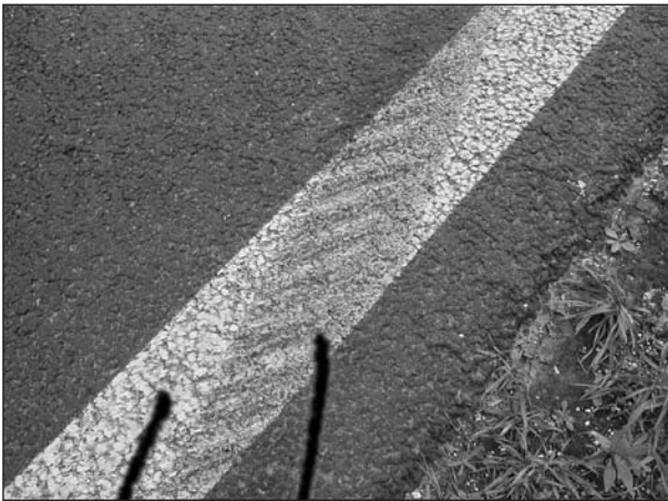
Fig. 5: Sliding marks
