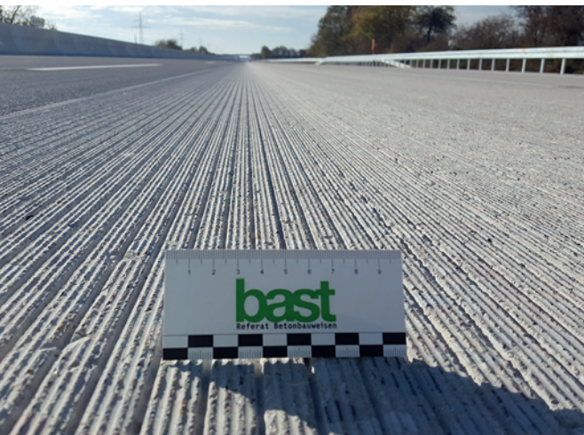
Road surface texture grinding: typ S+ 2.4/2.2 – 2.4/18
