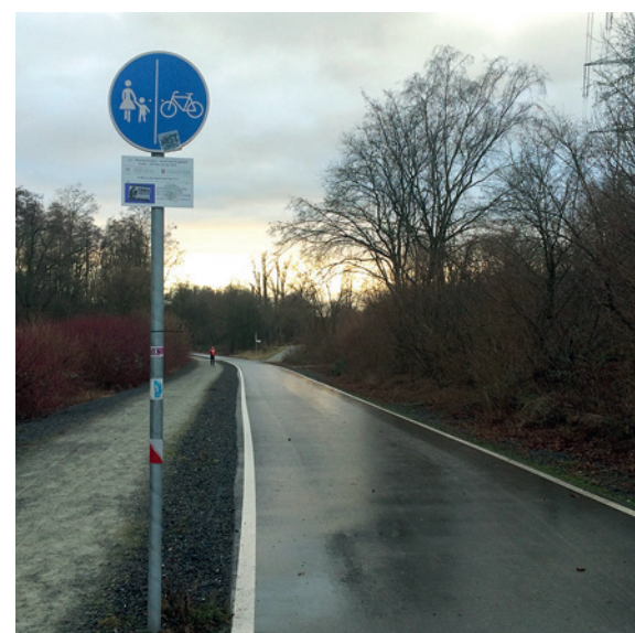
Section of a bicycle highway with a bicycle traffic space of four metres in width
