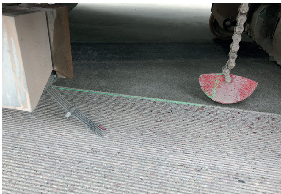
Laser-supported control of line alignment of grinding machine
