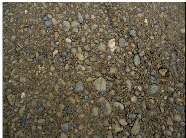
Fig. 2: Surface of the modified gravel base layer immediately after installation
