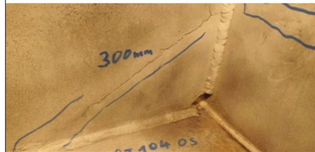
Fig. 5: Rheinbrücke Leverkusen (A1): cracks within the load application of the outer DS inside the box girder
