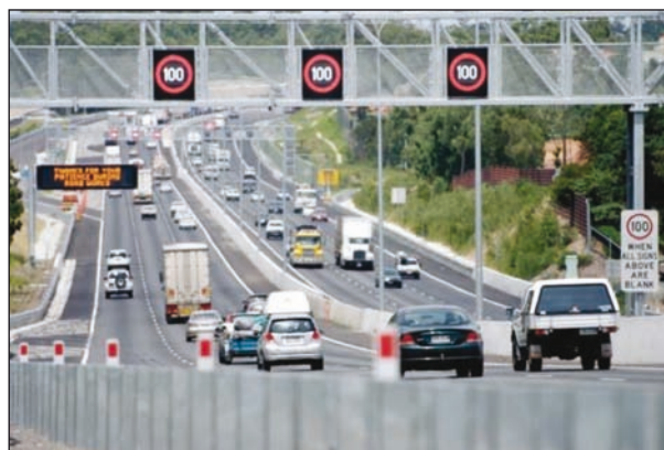
Bild 3.11: Variable Speed Limits and Lane Control Signs in Queensland Australien (entnommen QUEENSLAND GOVERNMENT, 2012)
